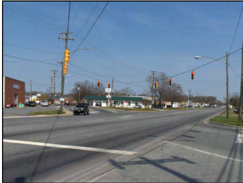
A lack of walkways and crossing points over Marshville's main roadway is a safety hazard.
