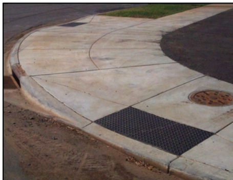
New sidewalks with ADA considerations.
