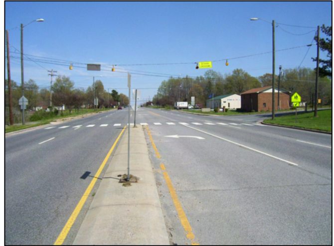
This turn lane is unnecessary since there is no roadway perpendicular to this intersection and could be converted into a landscaped pedestrian safety island.
