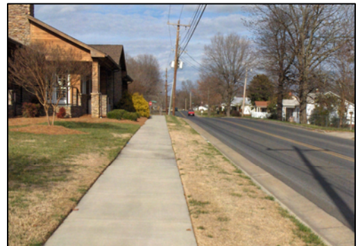
A new sidewalk to the library along Olive Branch Rd.
