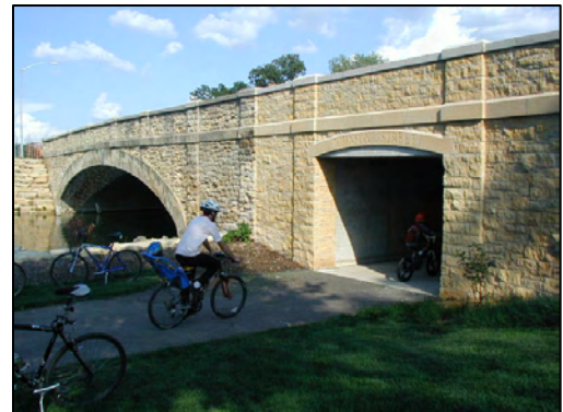
This underpass was designed and built during bridge construction
