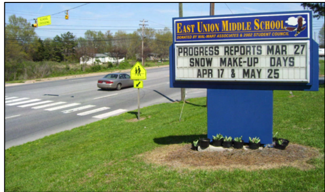
The only true access to East Union Middle School is by way of US 74. Note that the crosswalk in this photo leads to no sidewalk
