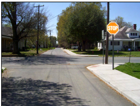
A new sidewalk on Church Street without a planting strip
