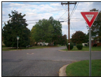
A four way yield intersection, with some modification, can become a mini-roundabout
