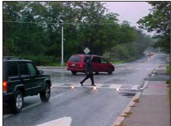
In-pavement flashing crosswalks improve visibility
