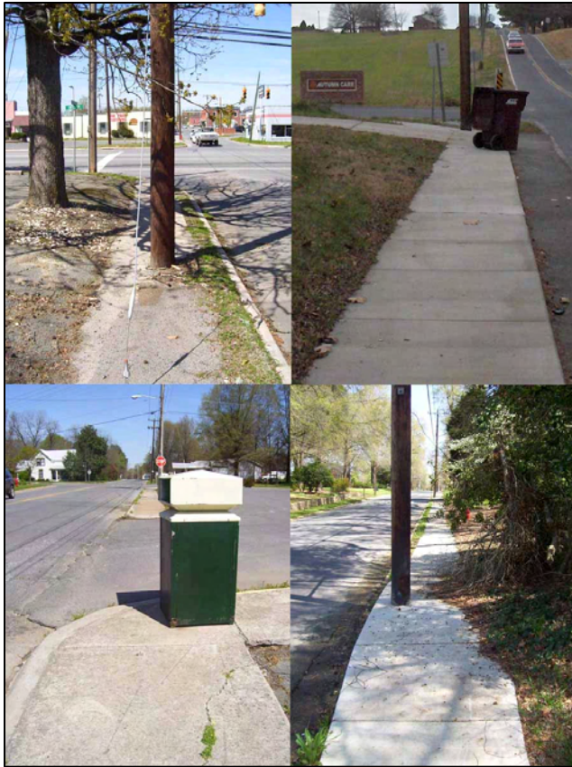
Most of the Town's sidewalks have inadequate space between the walkway and the roadway, allowing curbside obstructions to walking.
