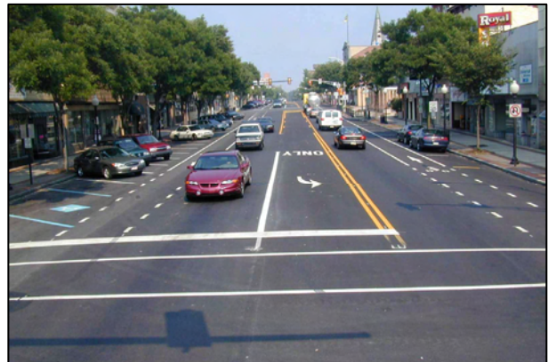
Back-in diagonal parking has benefits for pedestrians (Photo by Michael Ronkin)
