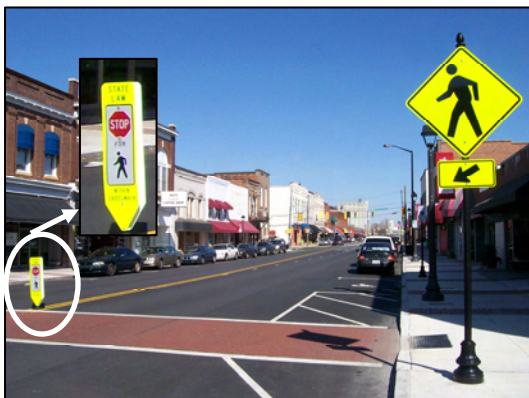
This crosswalk in Mooresville, NC uses a Pedestrian Crossing street sign, an in-street warning sign and pavement markers
