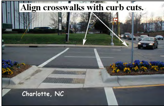
Although this crosswalk includes positive features such as a countdown signal, a pedestrian refuge island, and detectable warnings, it fails to line up with the curb cuts.
