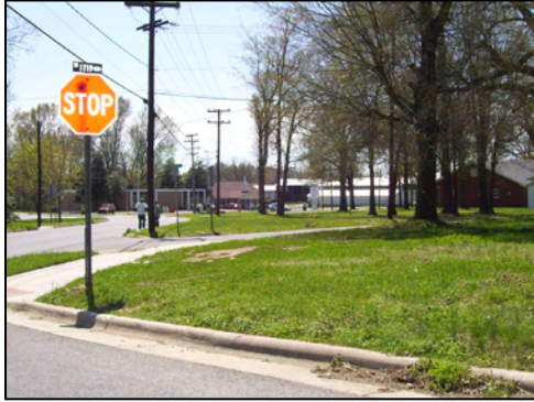
Connecting missing sidewalks links is a top priority.
