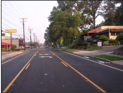
A lane conversion creates bike lanes from motor vehicle lanes and a new center turn lane.
