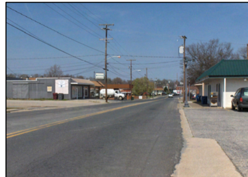
There are significant gaps in the sidewalk network
