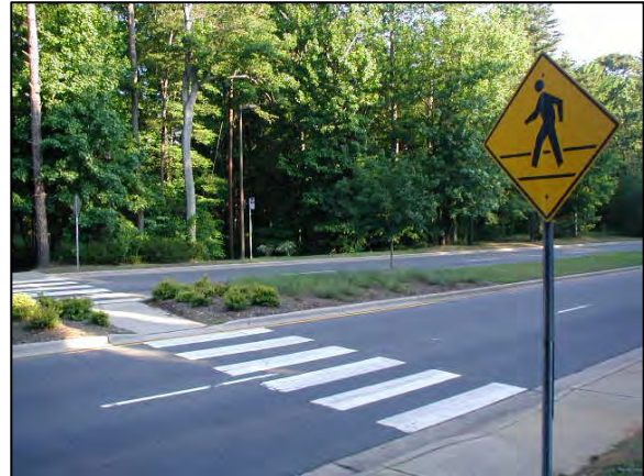
A Mid-block crosswalk in Charlotte, NC that has piano-style markings and a pedestrian refuge island
